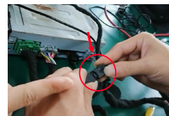
3. Connect CarPlay's LVDS cable with the original car head unit's video cable
